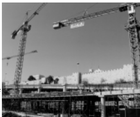
Bypass for the convenience of Jewish Settlers on what was Previously Palestinian Residential Area
